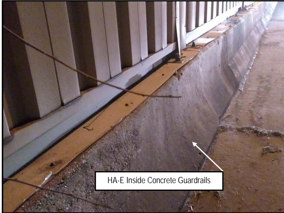
Photo 5: View of HA-E on the eastbound I-440 bridge over Lealand Lane
