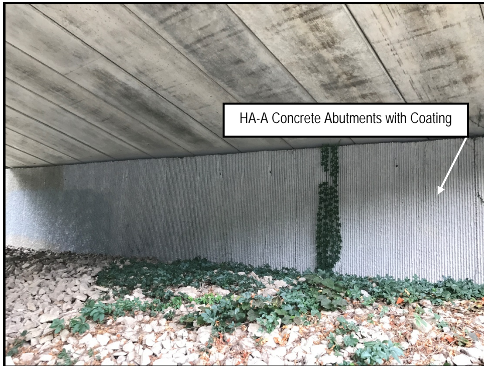
Photo 1: View of HA-A on the eastbound I-440 bridge over Lealand Lane
