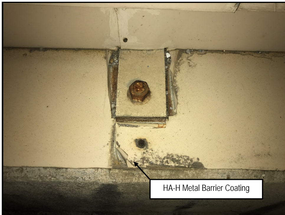
Photo 8: View of HA-H on the eastbound I-440 bridge over Lealand Lane
