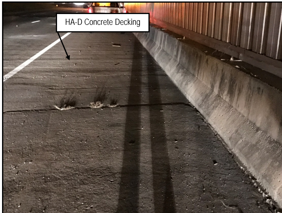
Photo 4: View of HA-D on the eastbound I-440 bridge over Lealand Lane
